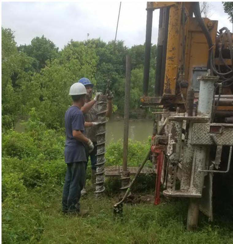
Adding an auger section (or flight) to the drill string. The smaller diameter drill rod is used to drive the drill bit at the bottom end of the auger.
