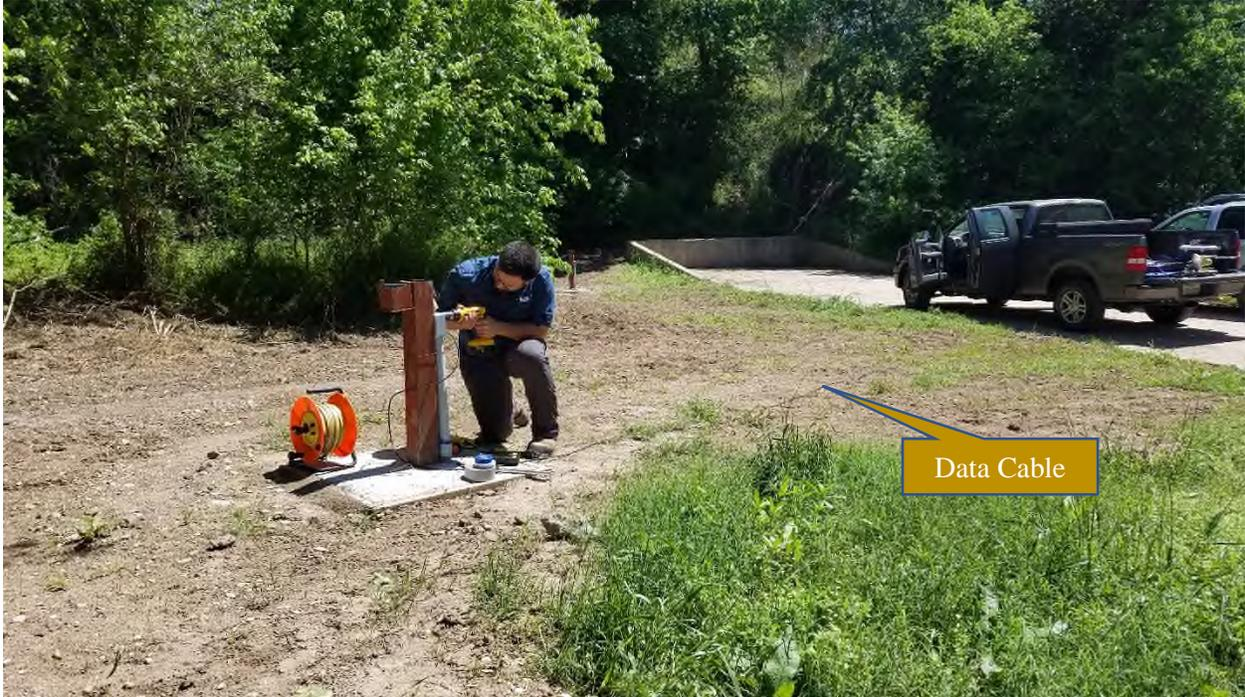
Additional above-ground conduits were installed at each well location to complete the installation of the transducer/telemetry system data cables. Monitor Well 1 is in the foreground and Monitor Well 2 is in the background.
