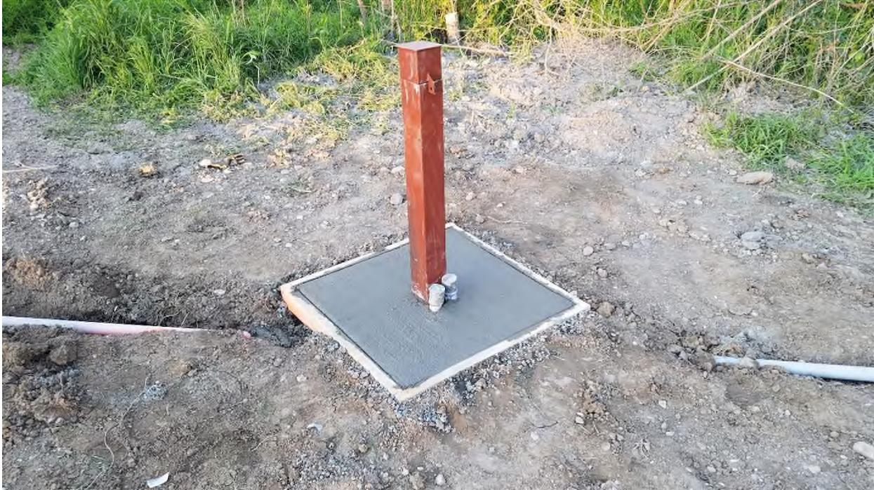
Monitor Well 2 after the concrete surface slab had been installed. The conduits for the transducer/telemetry system can be seen in the picture. The PVC conduits were buried below ground level for additional protection to the cables.
