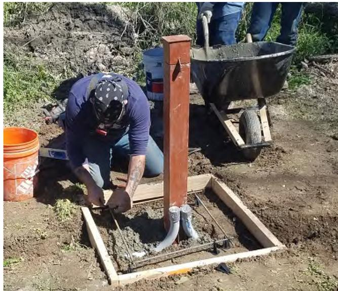
Each well then had a surface slab of cement installed and PVC conduit connections (grey pipe ends) for the transducer/telemetry system data cables. Monitor Well 2 is shown in this picture.
