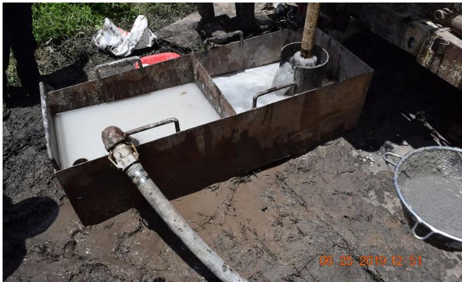
The drill rod passes through a pipe passing through the bottom of the trough on the right. The pipe is inserted in the borehole and the annulus is sealed using bentonite. This contains the water within the borehole and trough.
