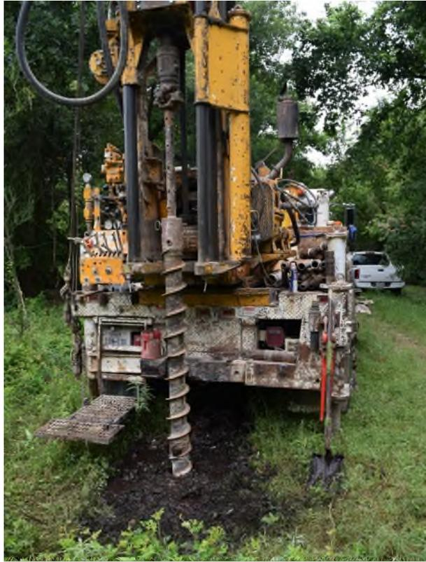
The additional auger flight and inner drill rod are connected to the drill rig and are ready to continue drilling operations.
