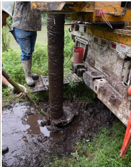
Drilling ahead with the auger rig. The rig had sufficient auger flights to drill to a depth of 55 feet below ground level. Drilling deeper than that required the use of mud rotary drilling methods.
