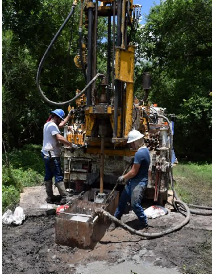
The auger rig is also capable of drilling using mud rotary methods using a small above-ground trough for the drilling fluid.
